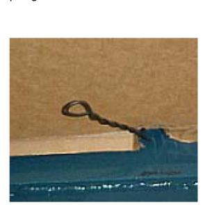
11. Wire from above needs to thread through this wire loop and be wrapped tightly.
