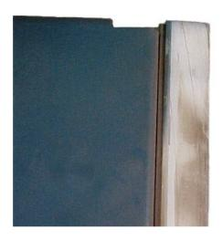
Use dry spray graphite on Vertical Plastic Runners (left photo) on each side of upper door.
